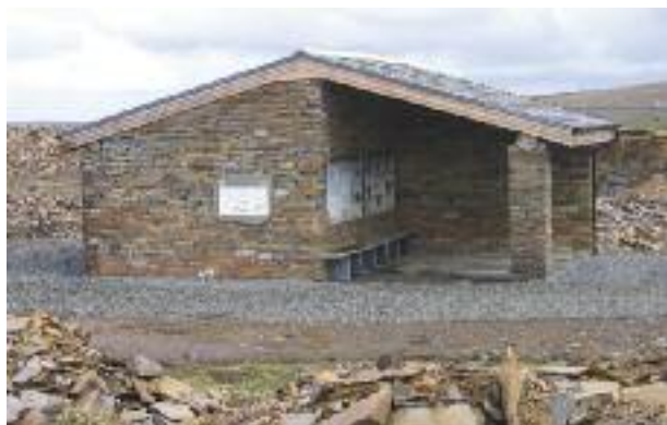
The new interpretative facility within Achanarras Quarry consisting of a flagstone visitor shelter and interpretative panels.
