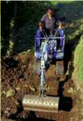
Excavation works at Tideswell Dale in 2003.
