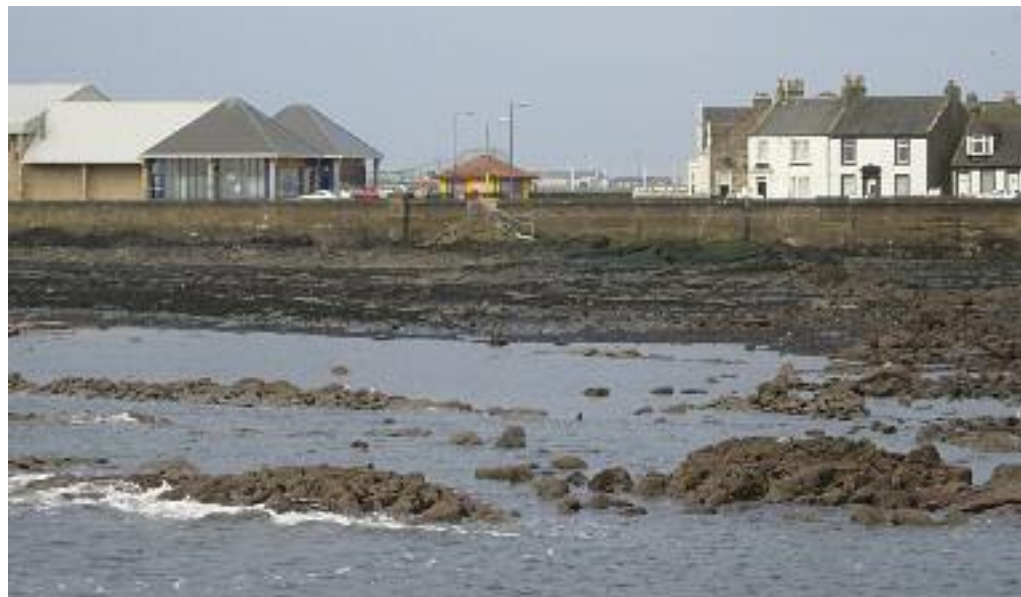
The seawall at Saltcoats Harbour and intertidal exposure before construction begins. Waves overtopping the wall here have flooded the town. All photos by Colin MacFadyen unless stated otherwise
